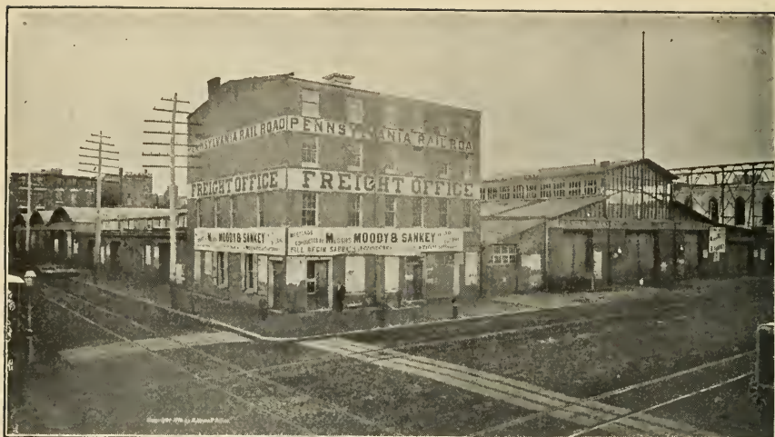
EXTERIOR OF OLD PENNSYLVANIA RAILROAD DEPOT, PHILADELPHIA.
